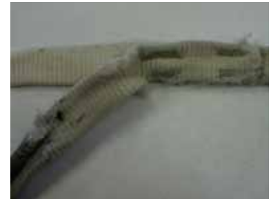
Badly worn Y-Line.
